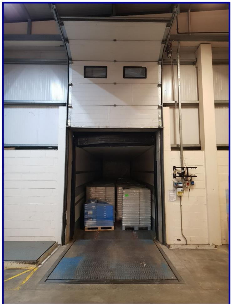
trols, dock levellers require experience based inputs at all stages of installation. Our engineering team are now regularly installing machinery from cutting out pits through to fitting final accessories such as wheel guides and safety lights, to commissioning controls and carrying out after-sales checks.
