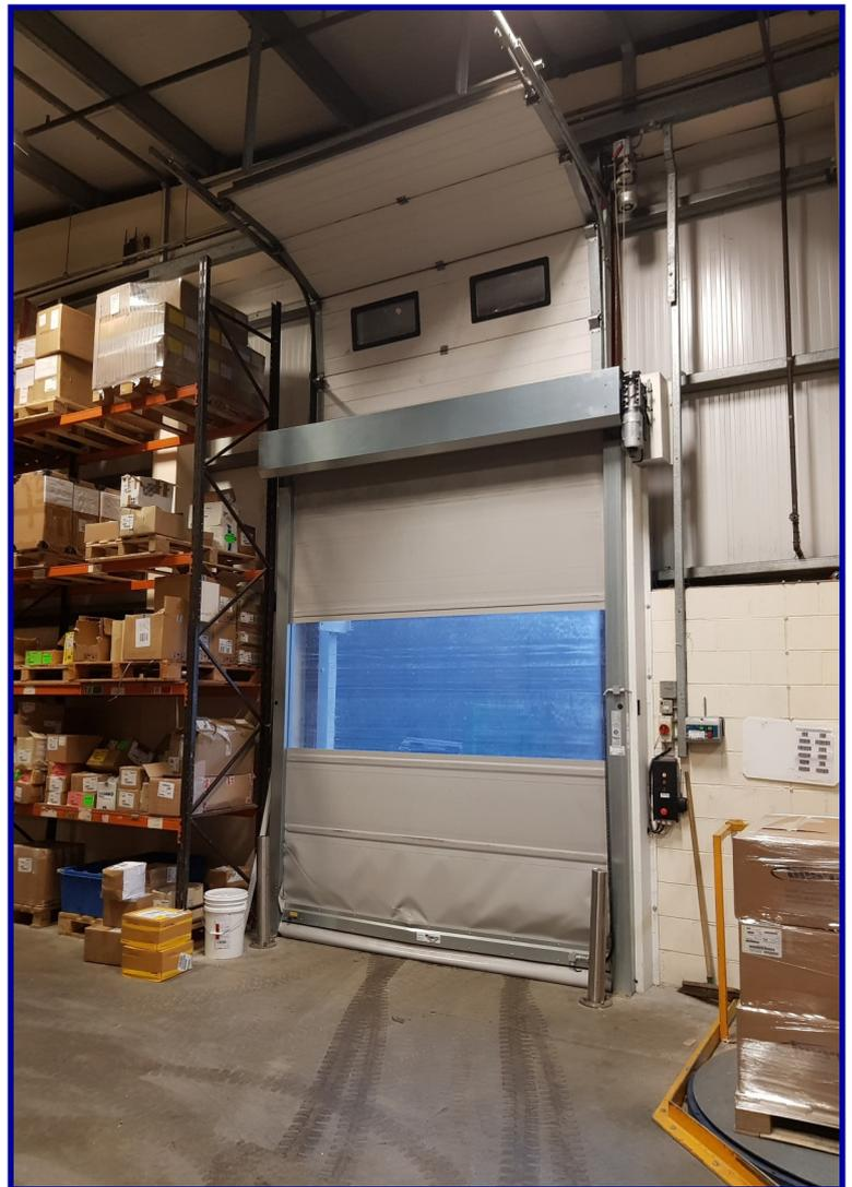
Pictured here is a combination solution of a Sectional overhead door [in the high *open* position] along with an automatically operated high-speed flexible door in the closed position preventing heat loss as well as prevent the entry of vermin and birds.
